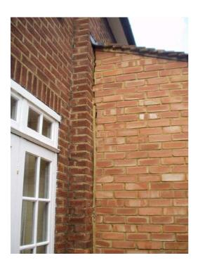
Above, a vertical crack between the extension and the rear house wall. There is further damage internally. Below numerically modelled soil suctions for the summer month, assuming a normal year. Bottom, right, a screen-shot of the disorder model.
